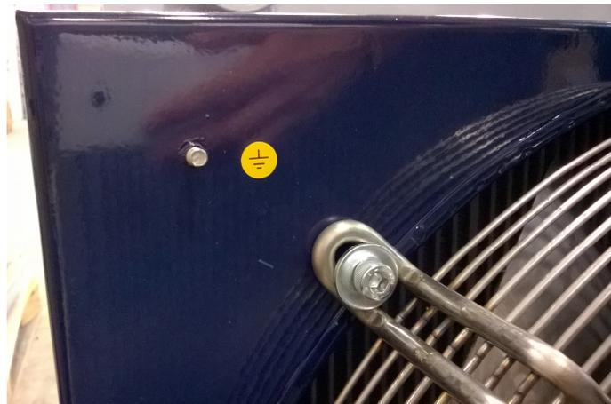
After having realised the connection, check the compliance of the intervention by measuring with a voltmeter/multimeter the actual value of the earth-heat exchanger resistance (which must be less than the value shown above) before attempting to operate the equipment.
